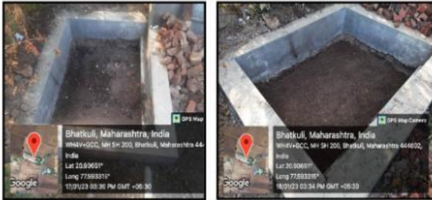
Rain water harvesting Pit
