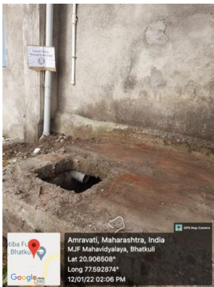
Liquid Waste Management Unit
