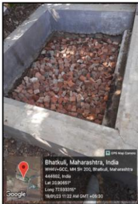
Sedimentary filling of Harvesting Pit
