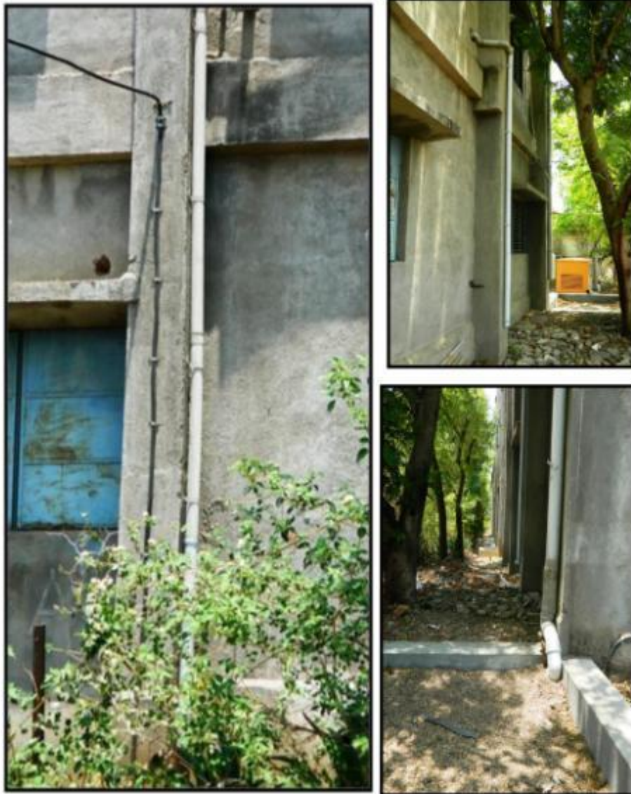
Water Harvesting pipeline network associated with common Pit
