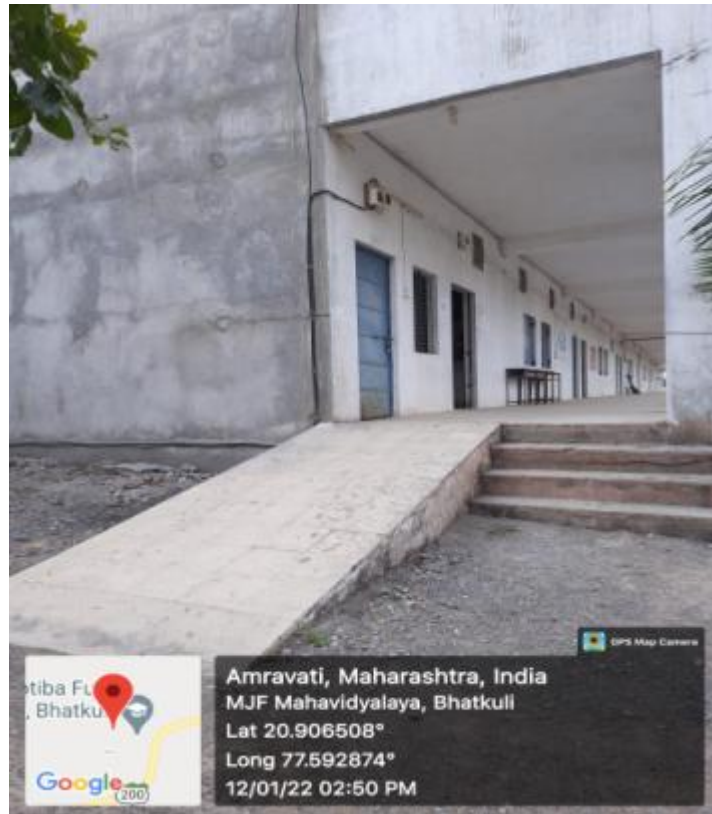
Ramp Facility for Differently Able Persons
