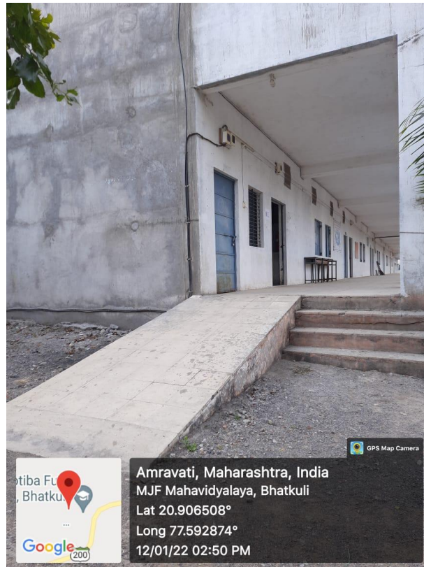
Ramp at Entry Point in Building
