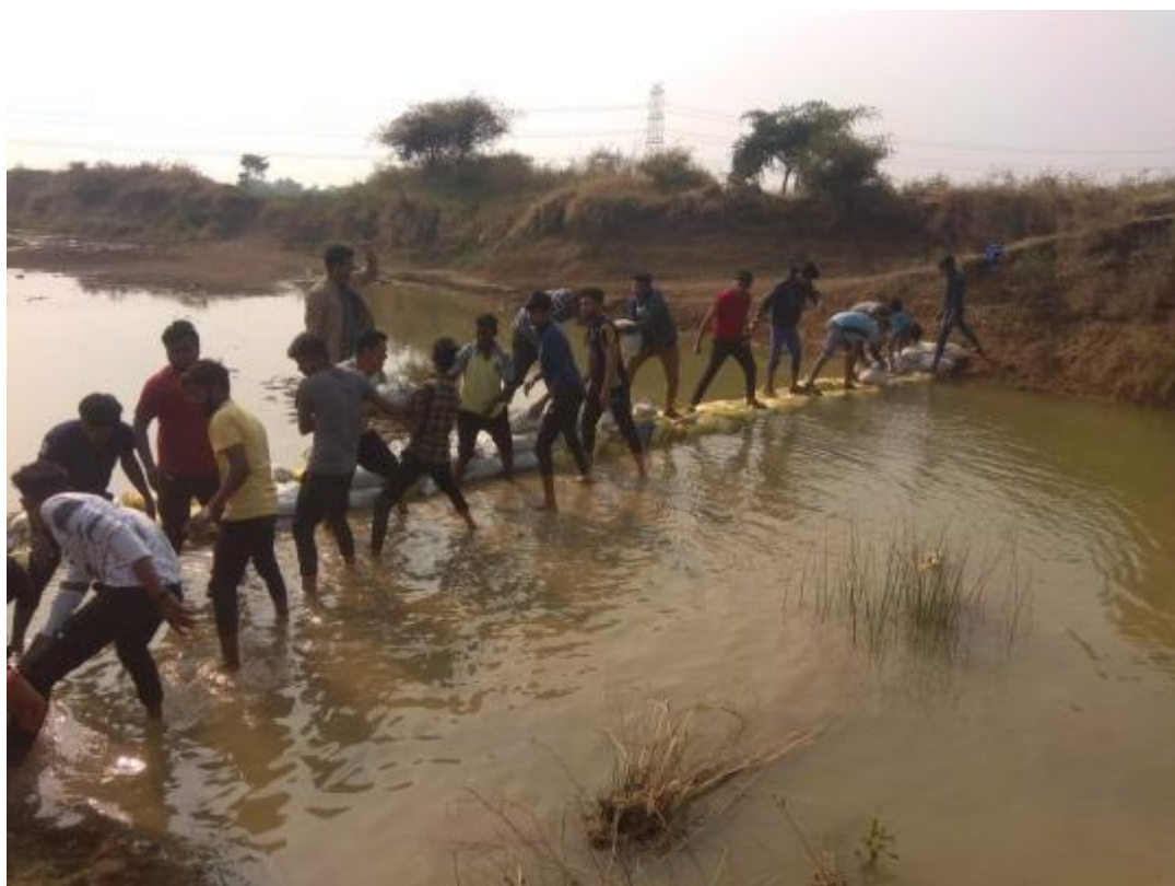
NSS volunteers working on temporary dam construction (Day 5; 23/01/2020)
