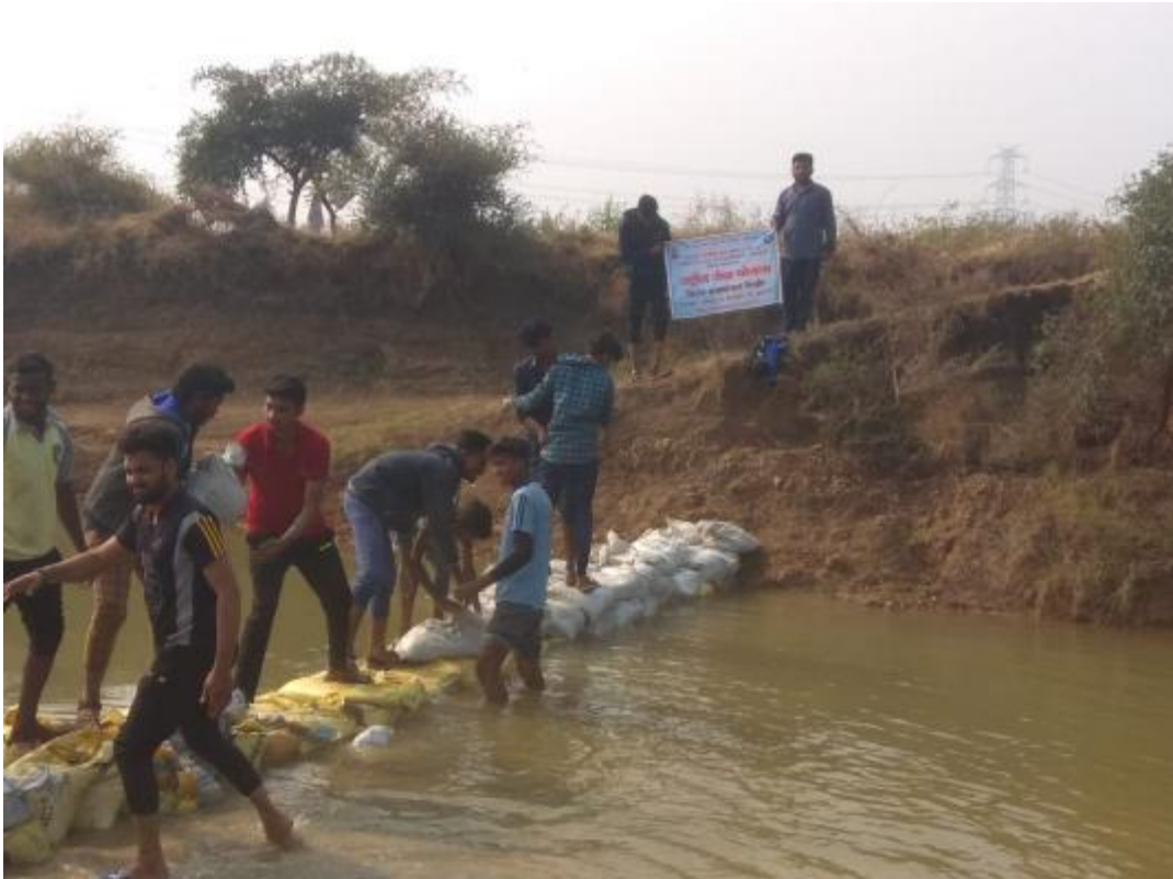
NSS volunteers working on temporary dam construction (Day 6; 24/01/2020)
