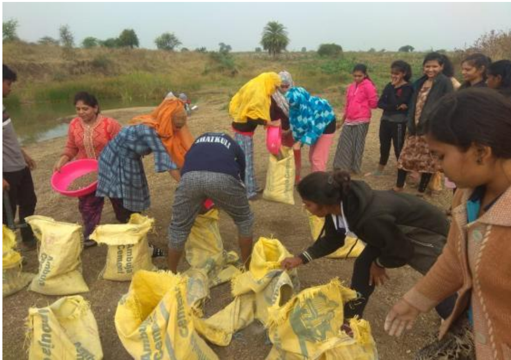
NSS volunteers working on temporary dam construction (Day 3; 21/01/2020)
